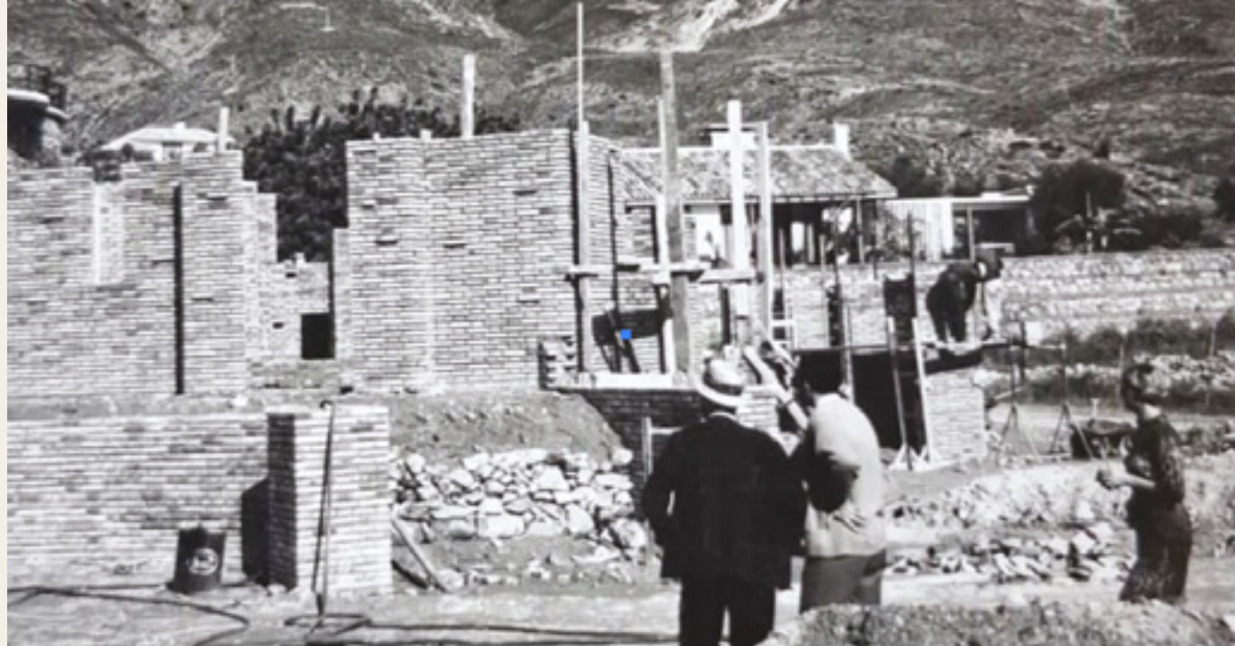
Robert Mosher observing the construction progress at Rancho Domingo in the 1970s.
